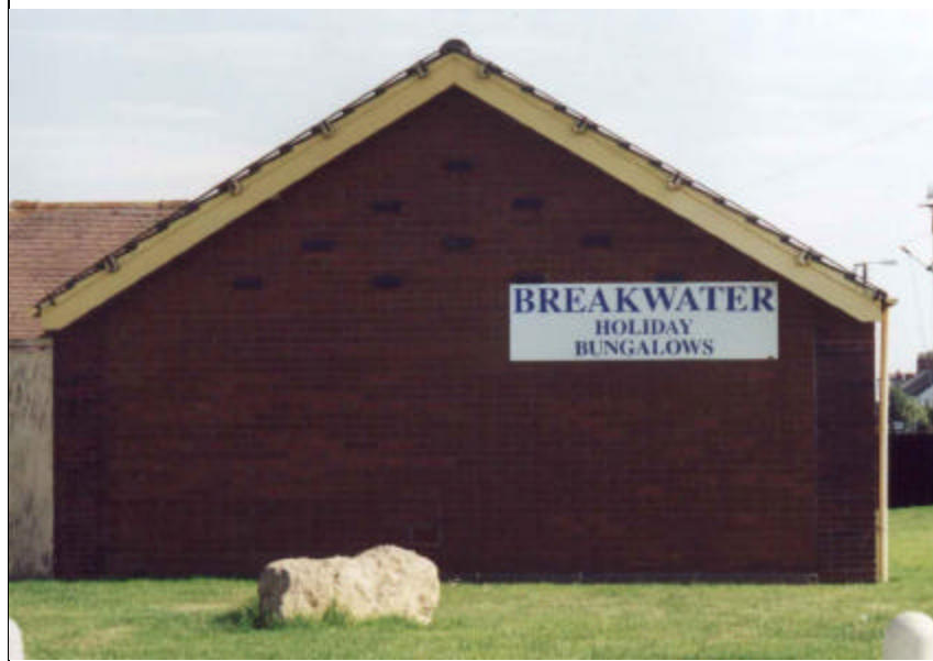
Figure 5: A recent development of bungalows with an ironic name sited just behind the sea defences near Trusthorpe between Maplethorpe and Skegness in eastern England.
